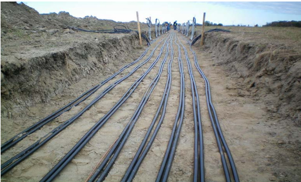
Photo Plate 12: Example of Cabling Being Installed in Trenches for Interconnection to Grid
