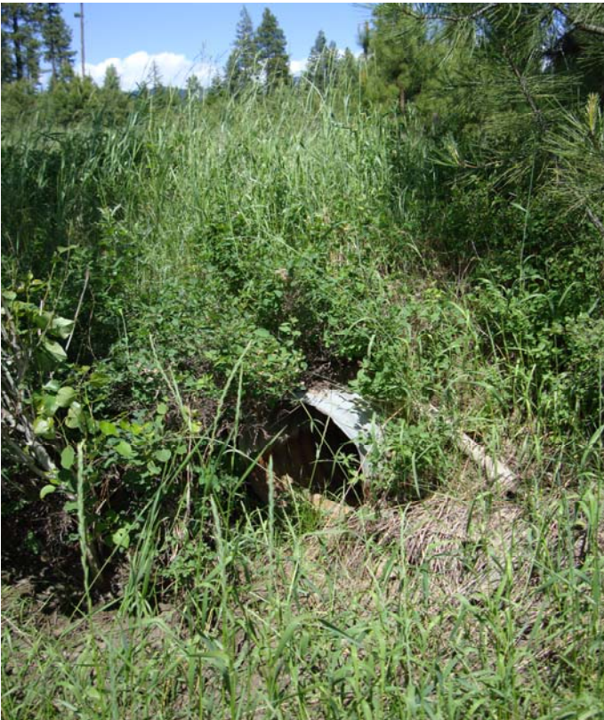
Photo 33: Stream S4 facing west (downstream) toward road culvert.
