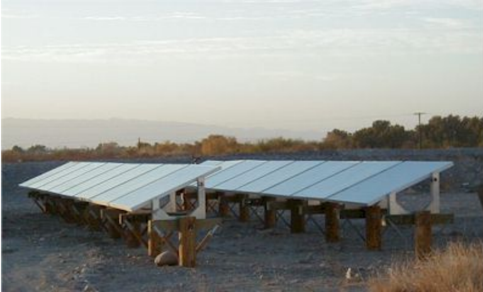
Photo Plate 7: Use of Timber Construction Materials in a Ground-Mounted Solar System
